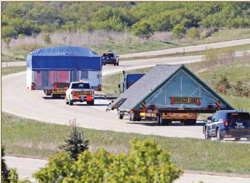
Moving the tavern to Old World Wisconsin required dividing the building into three pieces and moving it by truck to the new location where it would have to be reassembled.
