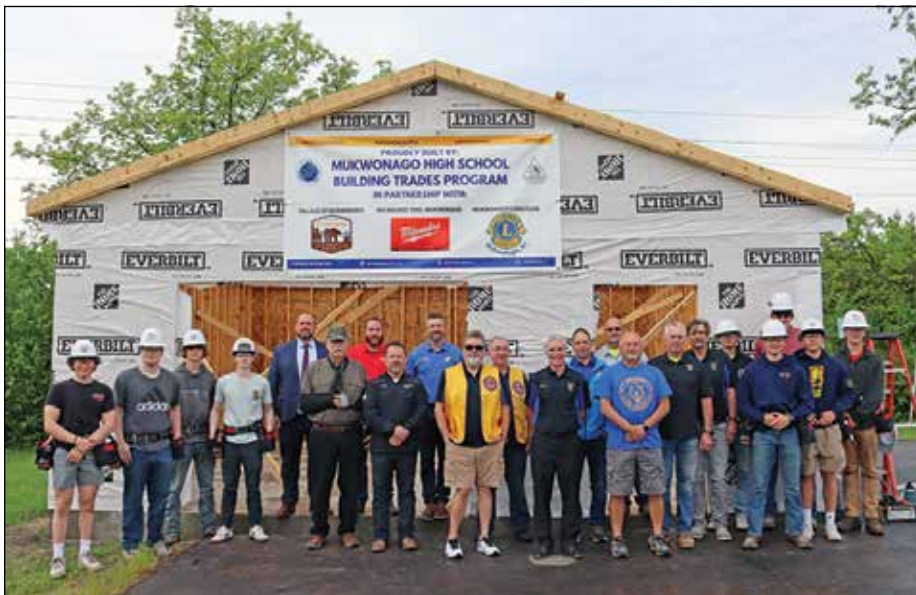
The entire crew that had a hand in the construction of a storage garage for use by local soccer teams at Miniwaukan Park gathers in front of the building. The project was a partnership between Mukwonago High School's Building Trades Program and the Village of Mukwonago, the Mukwonago Lions Club, and Milwaukee Tools of Mukwonago.
