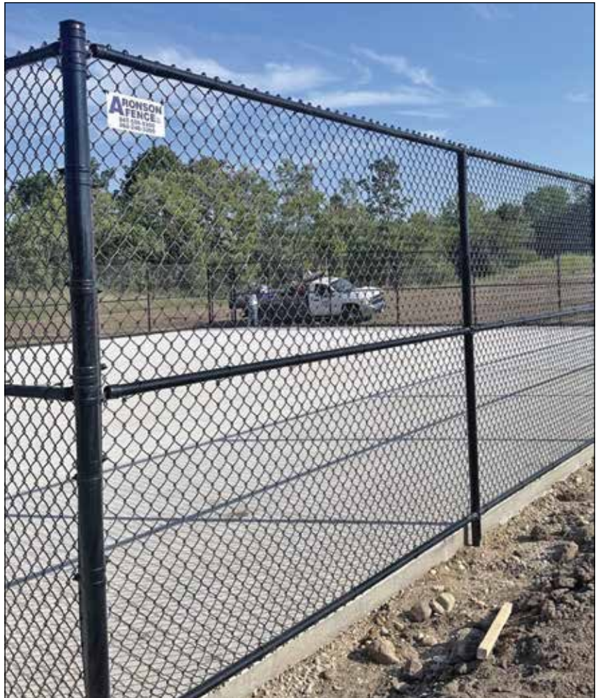
above: Chain Link Fences work well to enclose a tennis court. They keep the ball inside the court area and spectators on the outside where they can safely observe the game.
