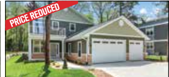
W5141 Plantation Rd, Elkhorn - Start your morning off with a cup of coffee on your private balcony off the master bedroom & end your day on the back patio. This home checks all the boxes, no need for updating here! Stunning New Construction 3 BR, 2.5 BA Lauderdale Lake Access, 2-Story Home w/partial water views. Open concept, main floor w/ Birch flooring featuring large eat-in kitchen with large island/bar, granite tops, SS appliance & pantry. Ample living area that leads to dining room overlooking the back yard with slider to paver stone patio. $864,900
