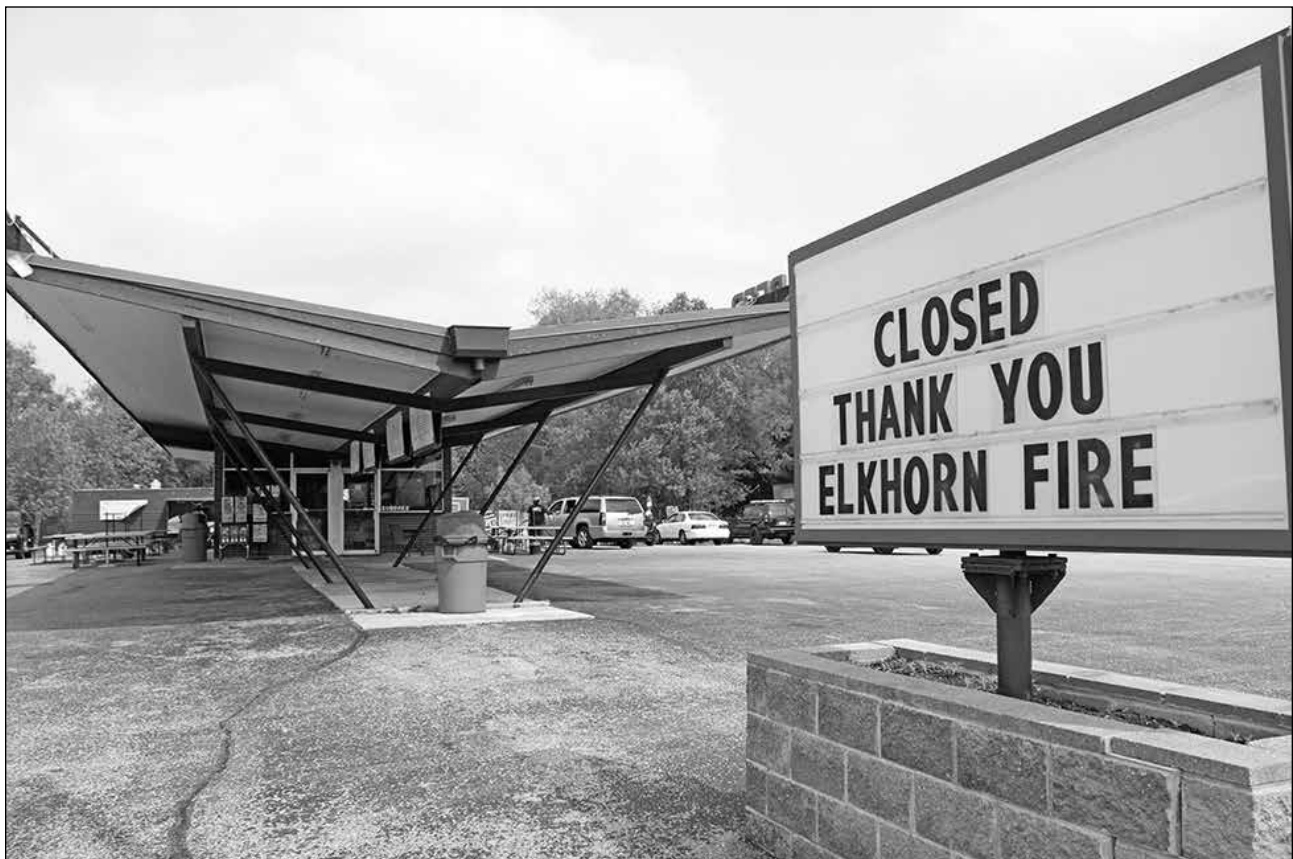
top: A fire after closing on May 18 has forced a temporary closing of Annie's Burger Town, a popular drive-in restaurant in Elkhorn. Boarded windows of the restaurant show where the heat from the fire blew out glass. above: A sign in front of Annie's expresses thanks for the Elkhorn Fire Department.
