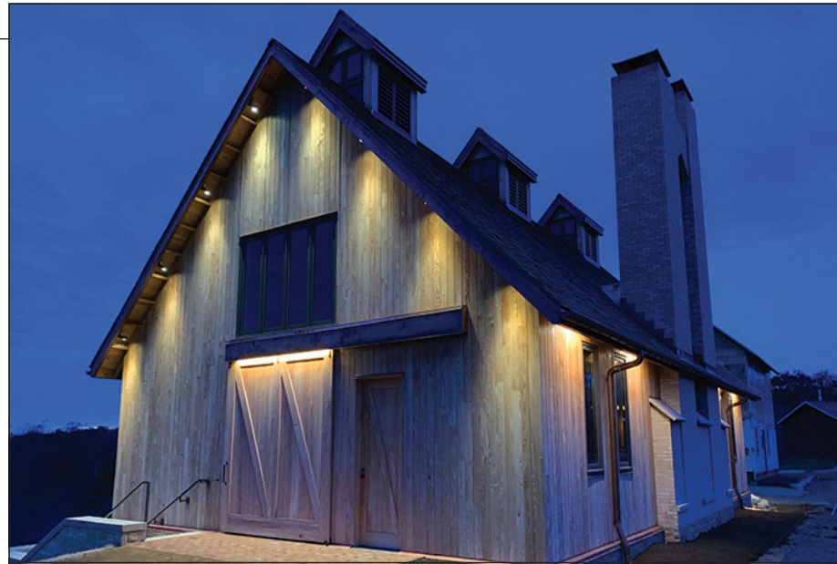
The recently completed brewing building at Old World Wisconsin historic site is shown lighted against the Wisconsin night sky. The building opened to the public this summer to share the brewing experience from the 1930s.
