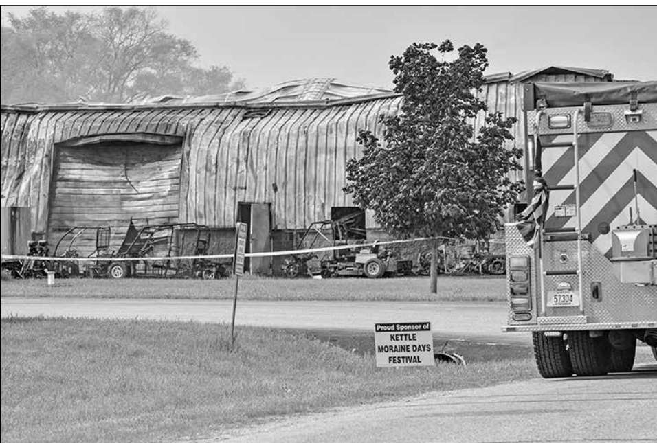
Summerset Marine Construction was severely damaged and several people were injured May 19 in the Town of Eagle.
