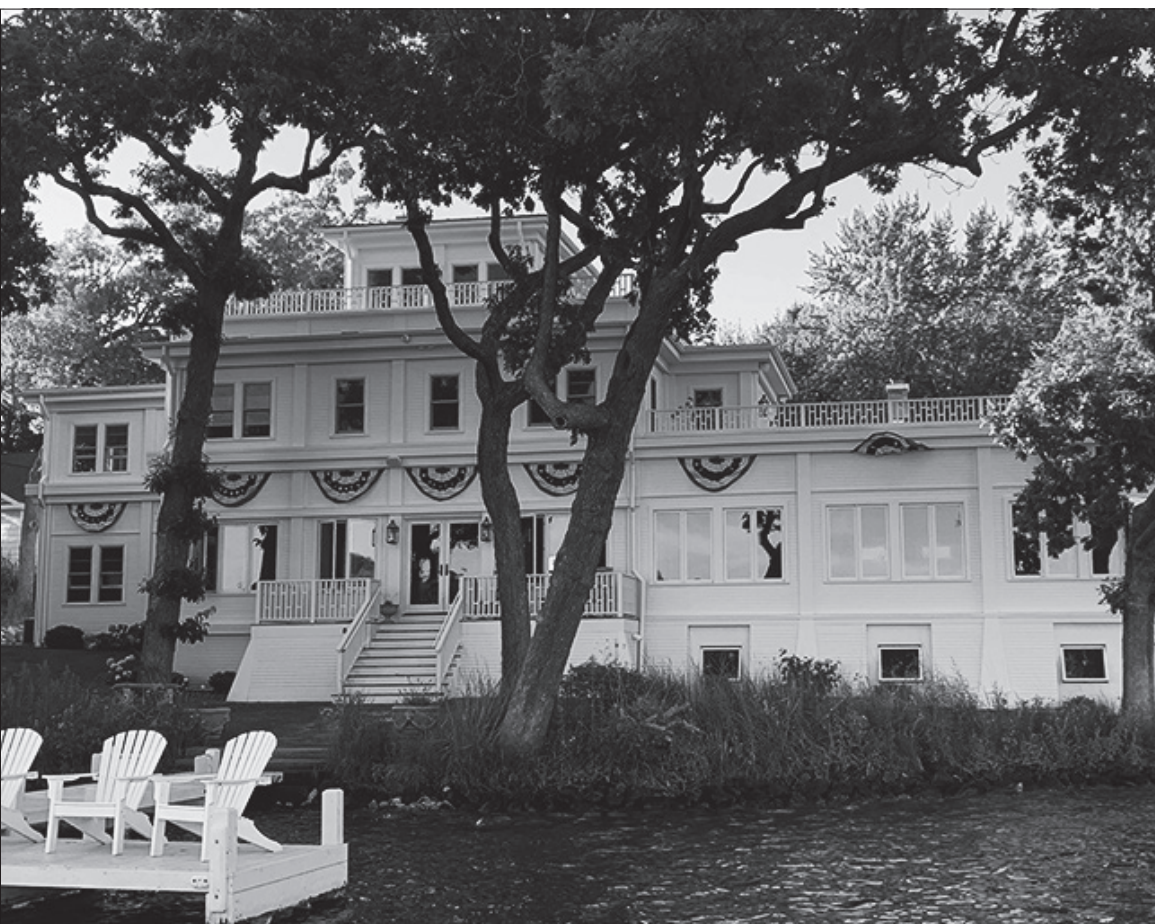
Jeffrey and Kelly Adams paid $1.22 million for this historic mansion at W5357 Lauderdale Dr. on Middle Lake. An Elkhorn contractor is accused of taking the couple's money for personal use.
