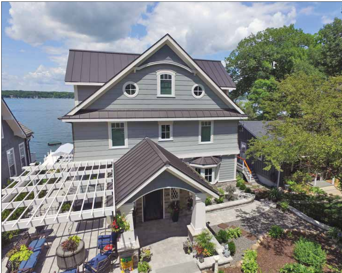
The award-winning remodel of a house on Geneva Lake by Stebnitz Builders included exterior work and a new second floor.
