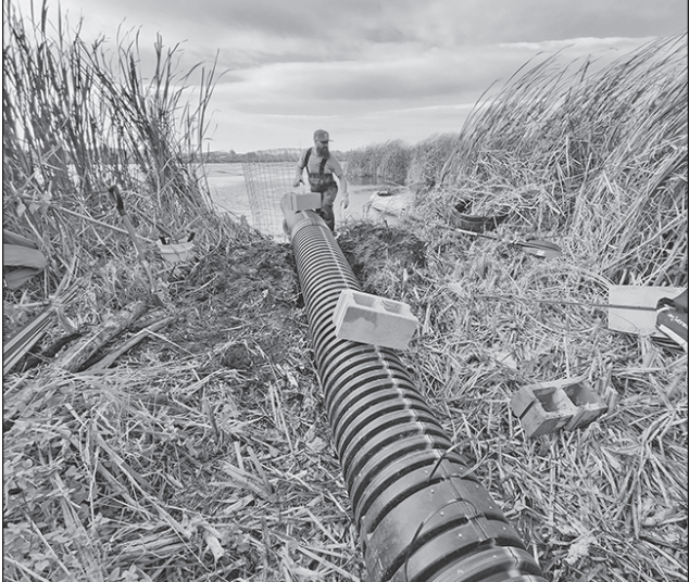
JOE TIMMERMAN FOR WISCONSIN WATCH Southern Lakes Newspapers Dan Fuhs, co-owner of Native Range Ecological, installs a pond leveler in October 2023, near the village of Rio.
